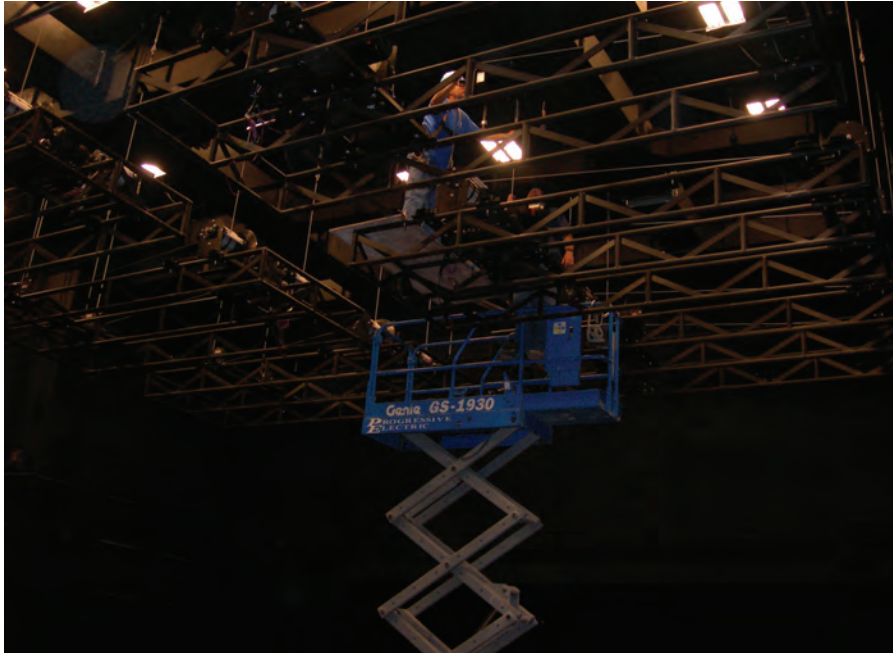
Workers install the new state-of-the-art lighting grid in the new studio theatre on May 23, 2007.
